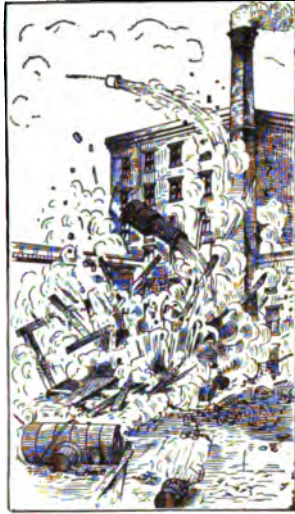
FIG. 157.—EXPLOSION OF BOILERS AT BROOKLYN, N. Y.
